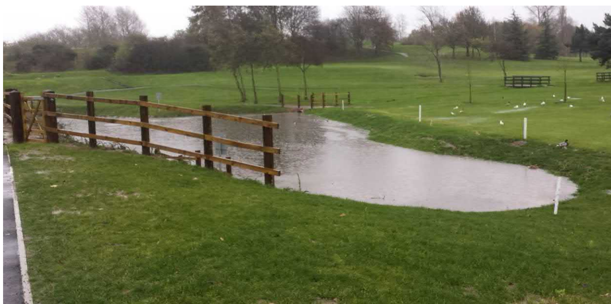
Figure 11: Existing Flood Storage Area nearing Capacity (November 2014)
